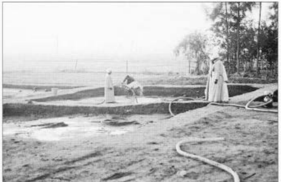
Figure 2 The shallow water table at Qantir.
