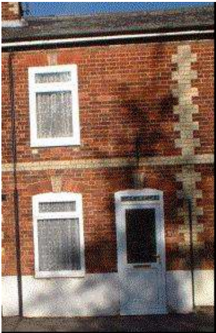
Figure 5. Front elevation of test house with new windows fitted.
