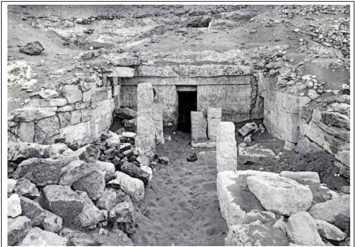
Figure 166. Tomb façade of Pepyankh the Middle (# 284), Meir D2 (after Blackman 1924: Pl. XXII).
