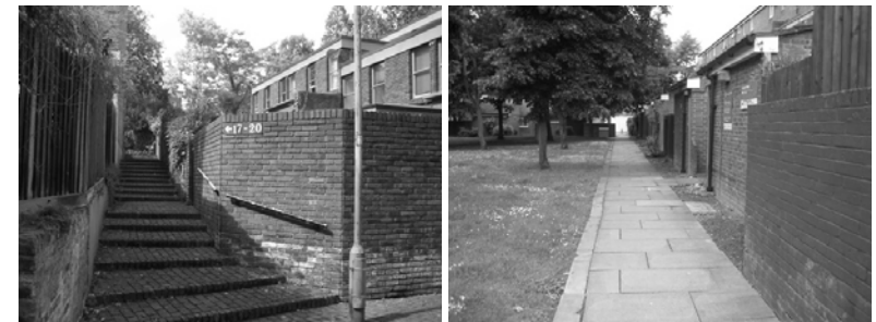
Figures 3 and 4: housing with high proportions of benefit claims located on low Choice segments, with no front doors facing the public domain and overlooking either a blank wall or a poorly-used public space.
