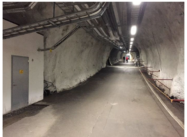
Figure 2. The “Svalbard tube”—the long entrance tunnel leading from the external concrete portal building into the mountainside to the three identical vaults. Photograph by the author. [This figure appears in color in the online issue.]
