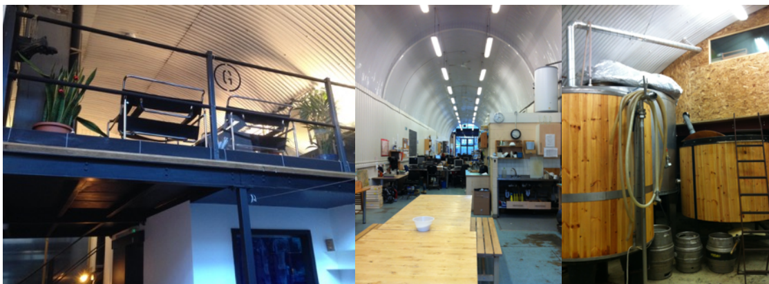
Figure 2: The interiors of three railway arches at a) FieldWorks, March 23 rd , 2017, b) Neal's Yard Dairy, 2013 c) London Fields Brewery 2013. © the author
