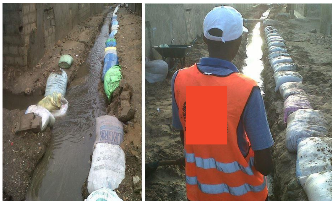
PICTURE 12: MANAGEMENT OF WATER IN TEMPORARY DRAINAGE CANALS SOURCE: CBO FACEBOOK PAGE UPLOADED IN SEPTEMBER 2013. ACCESSED ON 10.12.2016
