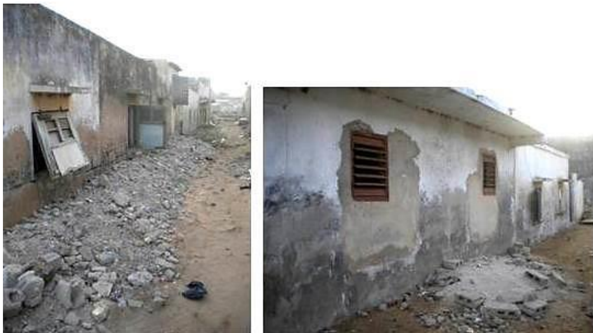
PICTURE 3: EXAMPLES OF REMBLAI IN DSM LONG PILES OF CONSTRUCTION WASTE ALONG THE HOUSE SERVE TO PROTECT THE BUILDING FROM EROSION CAUSED BY FLOODWATER. REMBLAI ALSO SERVES AS A DRY PASSAGE WAY. SIGNS OF CONSTRUCTION AROUND WINDOWS SHOW INCREMENTAL RAISING OF HOUSES: THE HOUSE IN THE BACKGROUND REMAINS AT ITS ORIGINAL HEIGHT. SOURCE: AUTHOR, JULY 2012
