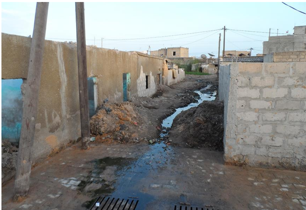
PICTURE 30: OPEN TEMPORARY DRAINS USED BY HOUSEHOLDS TO CHANNEL WATER IN GRN FROM UNSERVICED STREETS TOWARDS THE UNDERGROUND CANAL. SOURCE: AUTHOR, SEPTEMBER 2014
