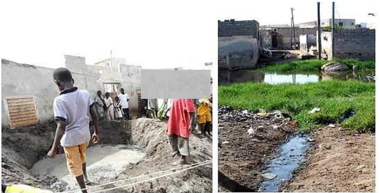
PICTURE 7: VIDANGE AND LEAKING OF BLACK WATER A LARGE VIDANGE HOLE DUG IN FRONT OF A HOUSE IN AN AREA SUFFERING FROM HIGH GROUNDWATER LEVELS. A STREET FLOODED BY GROUNDWATER AND ILLICIT SEWAGE LEAKS FROM SURROUNDING HOUSES. SOURCE: AUTHOR, APRIL 2015 & NOVEMBER 2014
