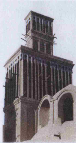
Figure 23, Badgir (wind tower) at Aqazadeh's house- Abarghu, Yazd. Source: http://www.yazd.com/album/017.htm . Retrieved 7.08.2005.
