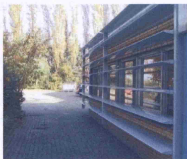
Figure 21 : Example of window shading with fixed horizontal louvres
