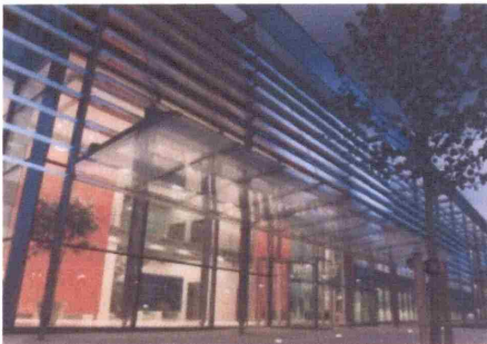
Figure 7: External shading examples, respectively: Solar fins- Cambourne Business Park, Cambridge, Membrane Louvre-Baader Bank, Germany, Brise Soleil- Addison, Wesley Longmans, Harlow [source: The Colt Group]
