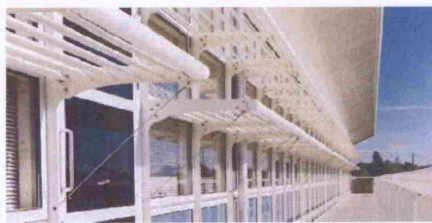
Figure 20 : Example of window shading with fixed overhang
