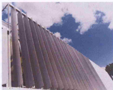
Figure 22 : Example of window shading with vertical louvres
