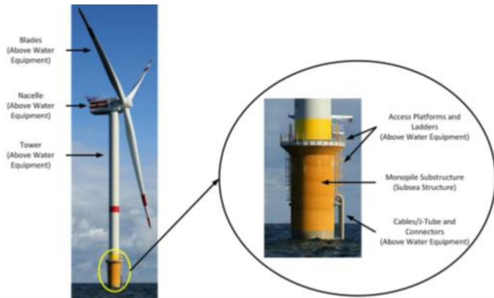
Figure 2-2. Different components of a typical offshore wind turbine mounted on monopile foundation (Sheppard and Puskar, 2011)
