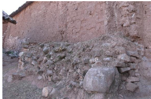
b) Base course of collapsed buttress B4 and B5
