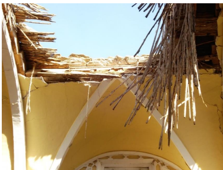
Figure 6.36 Failure of the composite layers after the 2007 Pisco Earthquake (courtesy of Erika Vicente)
