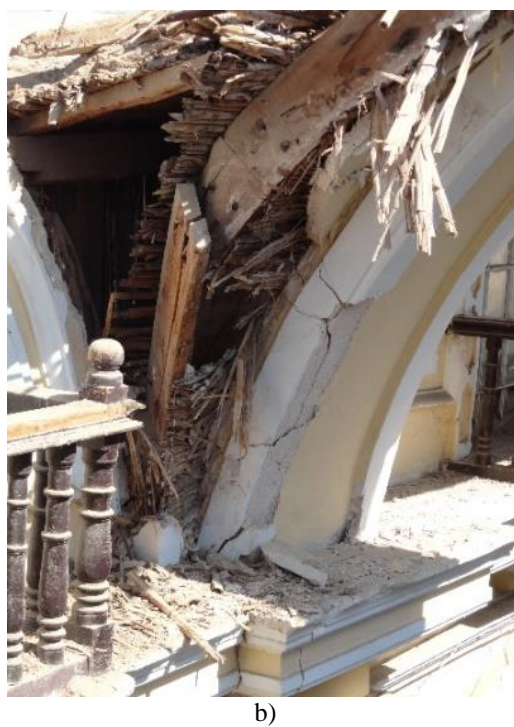
Figure 4.43 Failure of the bay-edge arches of bay 2: a) partially collapsed arch at the Eastern end; and b) failure of the nailed connections near the spring point of the arch at the Western end
