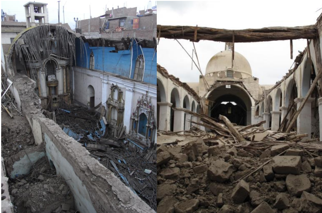
Figure 1.4 Examples of planked timber vaults that collapsed during the 2007 Pisco earthquake
