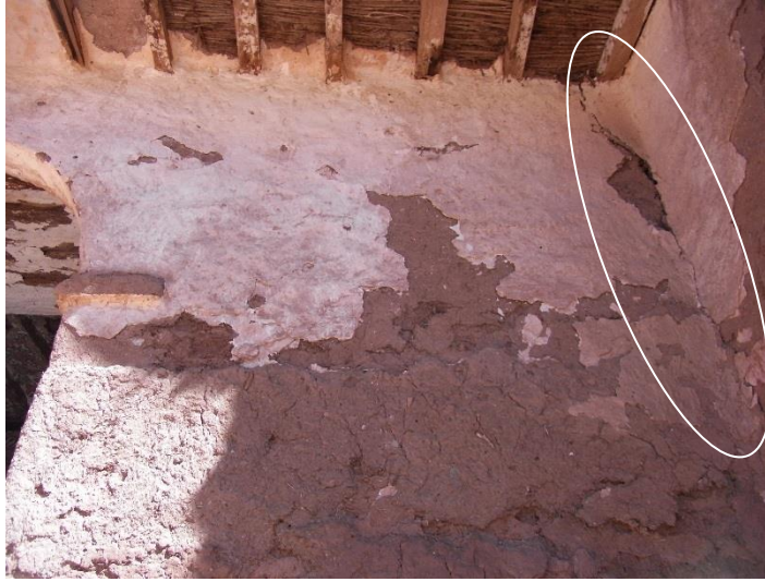
Figure 5.2 Crack at the interface WI.1/WI.4
