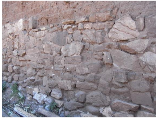
Figure 7.20 Rubble stone masonry of the base course of the Church of Kuño Tambo
