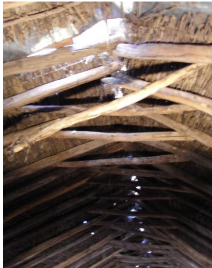
Figure 7.18 Connection between rafters and connection of collar beams to rafters
