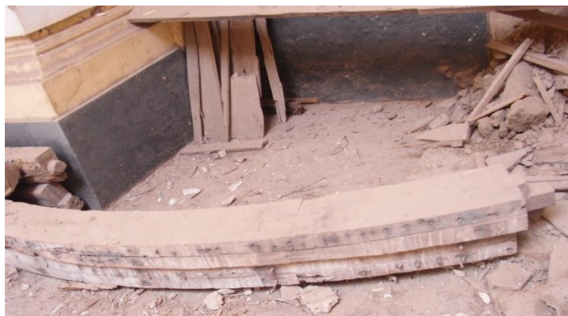
Figure 6.35 Collapsed internal arches on the ground of the Cathedral of Ica, showing that the canes were fixed to only one alignment of planks in each arch
