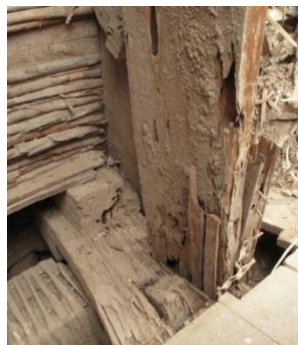
Figure 7.52 Deteriorated secondary arch (Credits: GCI)
