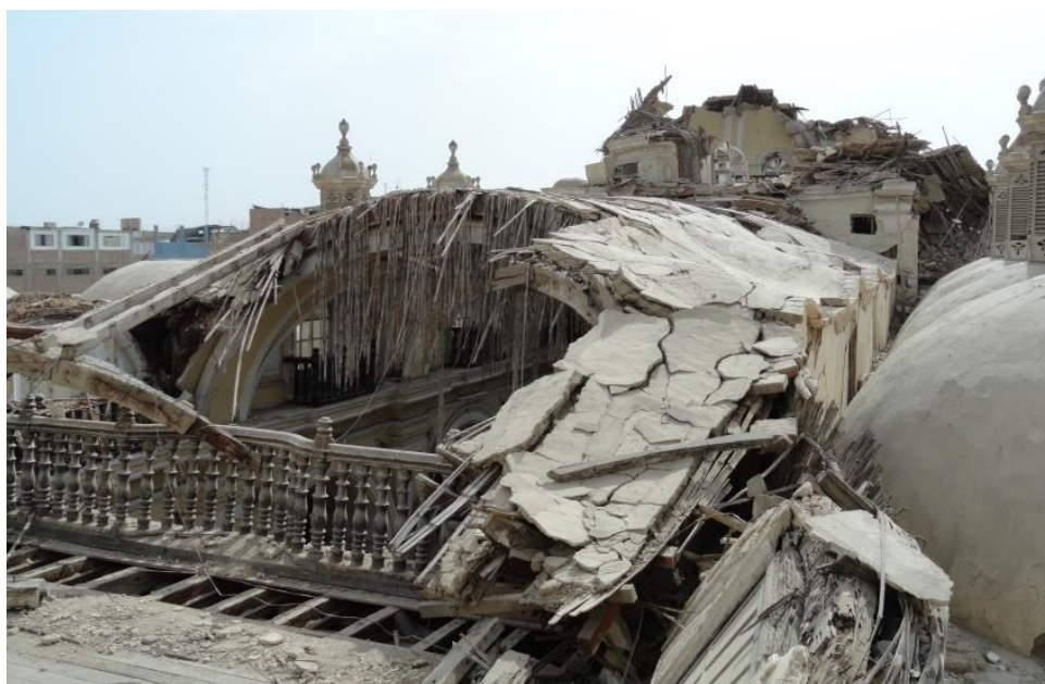
Figure 4.42 Damage state of the timber vault and principal dome of the Cathedral of Ica in 2011 (courtesy: Erika Vicente, PUCP)
