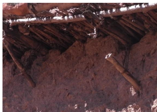
a) Wooden confinement elements in the Church of Kuño Tambo
