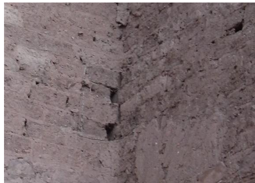
c) Interlocking of units between buttress B12 and wall W1.4
