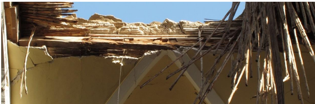
Figure 7.31 Splitting of the beam at the top of lunettes
