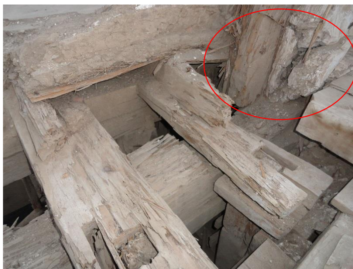
Figure 7.46 Poor construction quality: connection of a lunette's arch to a longitudinal beam in bay 2 (courtesy of Erika Vicente, PUCP)
