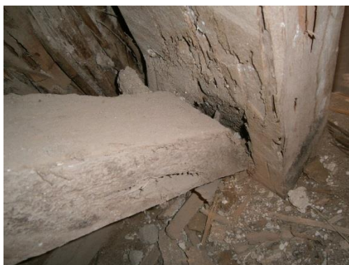
Figure 7.44 Withdrawal of a nail in the Cathedral of Ica without splitting of the timber members (courtesy of Erika Vicente, PUCP)
