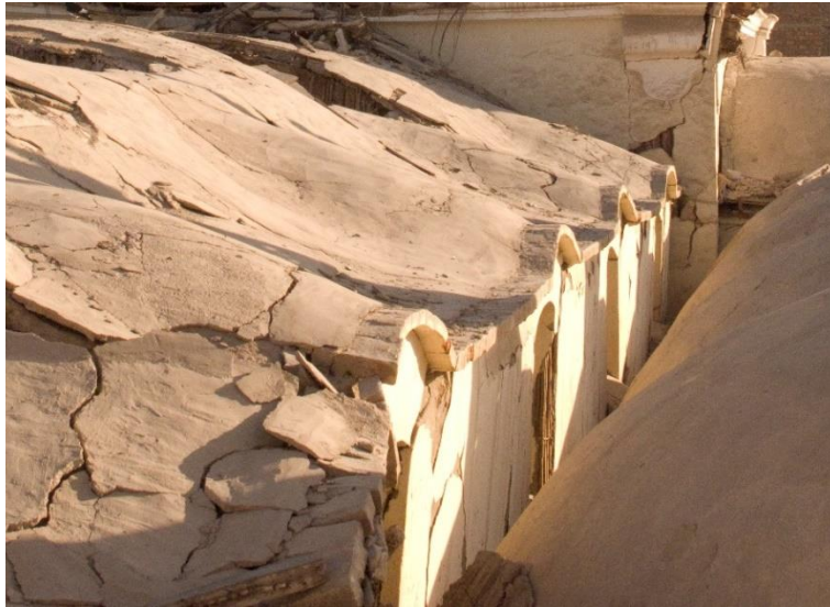
Figure 6.32 Generalized cracking of the roof of the Cathedral of Ica (courtesy of Claudia Cancino)
