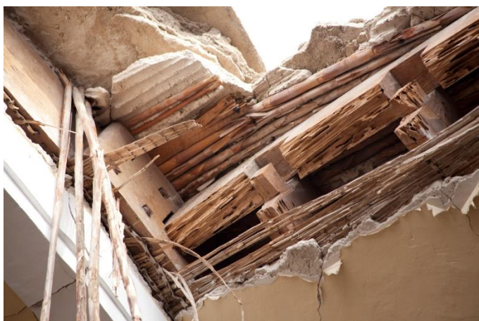
Figure 4.41 Failure of the mortice and tenon connection at the top of lunettes (courtesy: GCI)
