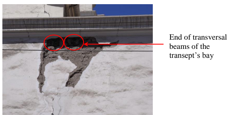
Figure 4.38 Damage on the North longitudinal wall, where it can be seen the end of the transversal beams of the transept bay
