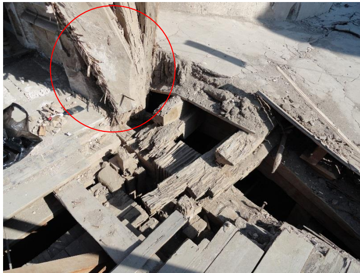
Figure 7.47 Poor construction quality: connection of a diagonal to a bay-edge arch in bay 2 (courtesy of Erika Vicente, PUCP)
