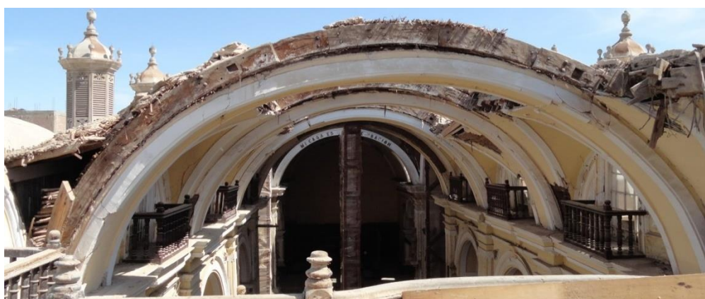
Figure 4.34 Representative bay-edge arch of the Cathedral of Ica (courtesy of Erika Vicente, PUCP)
