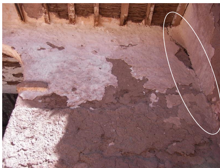
Figure 7.14 Crack at the interface WI.1/WI.4
