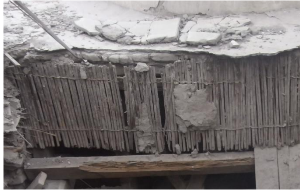
Figure 6.34 Cane system of the Cathedral of Ica's roof
