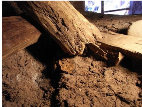
Figure 7.17 Detail of connection of rafter to wall-plate in the nave
