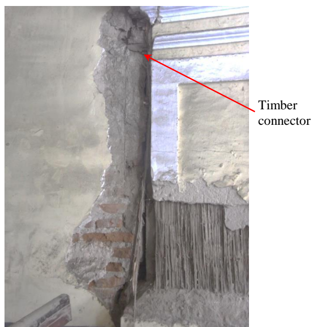
Figure 4.39 Timber links between a lateral pillar and the North longitudinal wall
