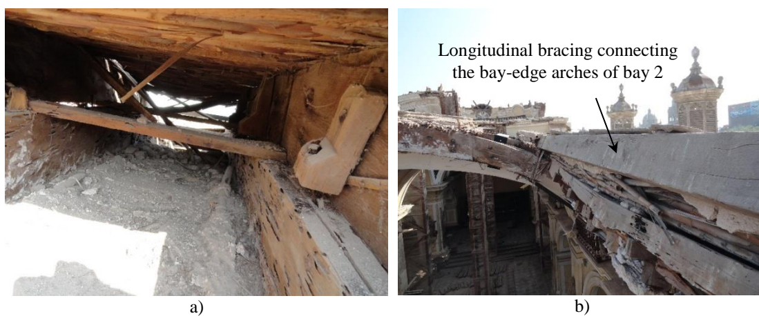
Figure 4.35 Longitudinal bracing of the timber vault of the Cathedral of Ica (courtesy of Erika Vicente, PUCP): a) connection of the bay-edge arches of adjacent bays; and b) connection of the bay-edge arches within each bay
