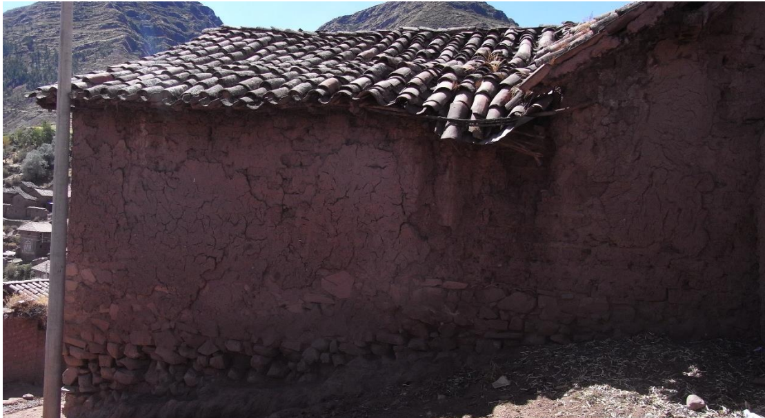
Figure 7.12 Deteriorated plaster in WL3
