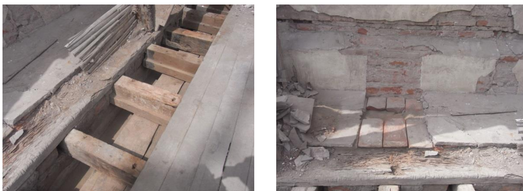
Figure 4.37 Choir loft's joists sitting on the façade
