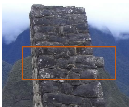
d) Confinement elements made of stone in Machu Picchu, Peru
