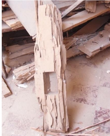
Figure 7.50 Deteriorated portion of top of lunette's beam
