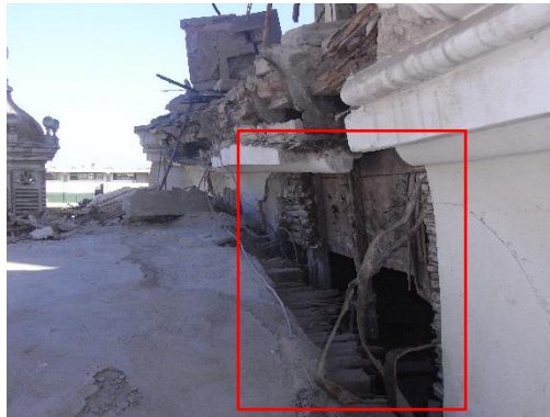
Figure 7.49 Damage caused by the interaction of bay 5 with the central dome's bay during the 2007 Pisco earthquake
