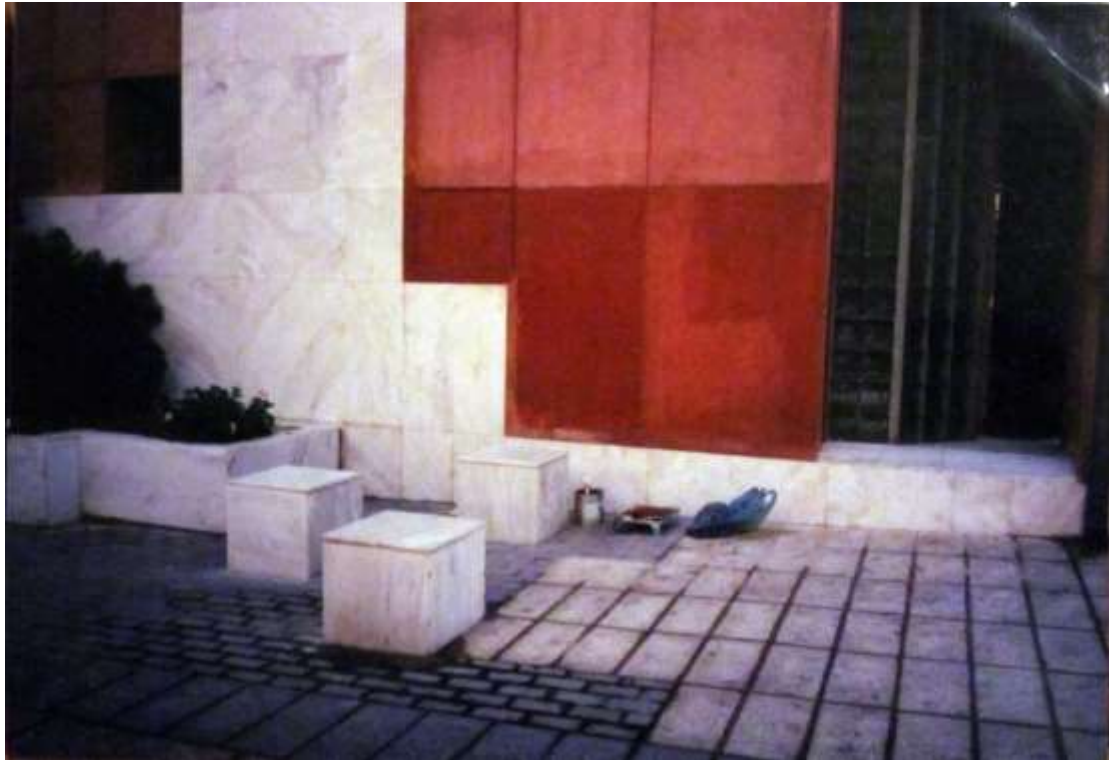
Figure 4.53 Different tiles that were eventually used for the public pavement meant that Suzana and Dimitris Antonakakis' original intentions could not be fully realised (Rhodes Urban Planning Agency Archive). The white marble used by the local construction crew used for the lower part of the exterior wall was supposed to match the material used for the public pavement. This design detail was meant to intensify the public character of the building.
