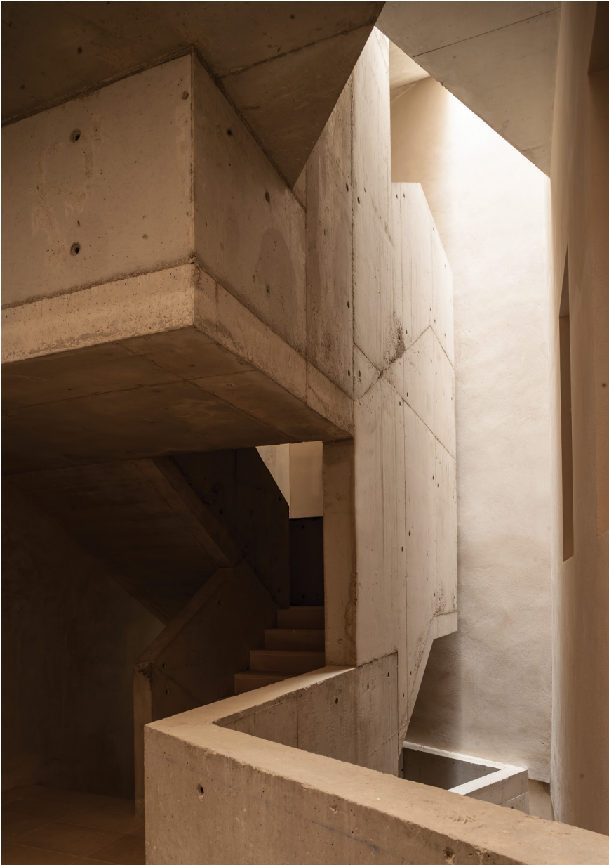
Figure 6. Flores Prats. Casal Balaguer (2009–). View into new circulation, balconies and light well. Photograph Adrià Goula.
