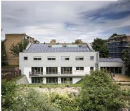
Figure 1: Mildmay community centre after the Passivhaus retrofit
