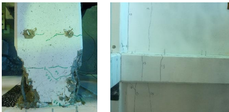
Fig. 5. Final damage state in C1; left: superior column, right: beam underside
