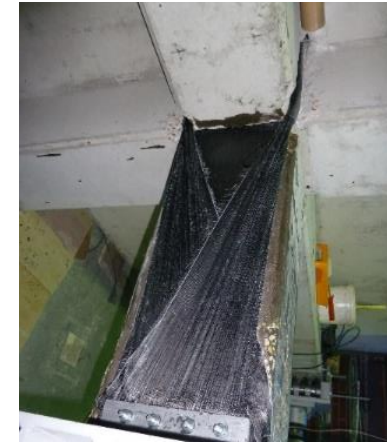
Step 7: Application of strips of FRP for shear strengthening and anchorage in beams; additional anchorage with bolted steel plates
