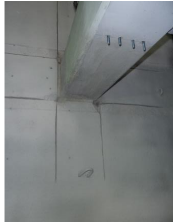
Step 6: Strengthening of beams and joint with FRP strands
