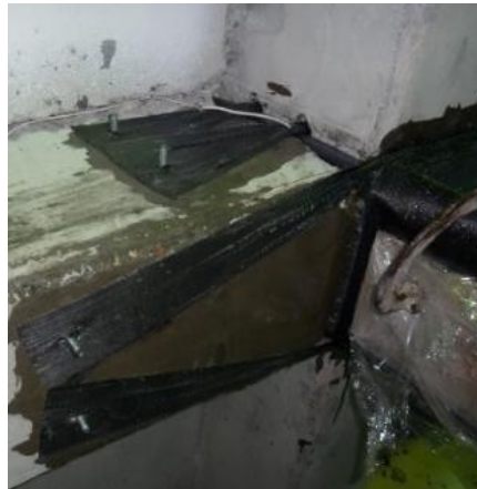
Step 6: Strengthening of beams and joint with FRP strands
