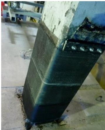
Step 5: Column confinement and shear strengthening
