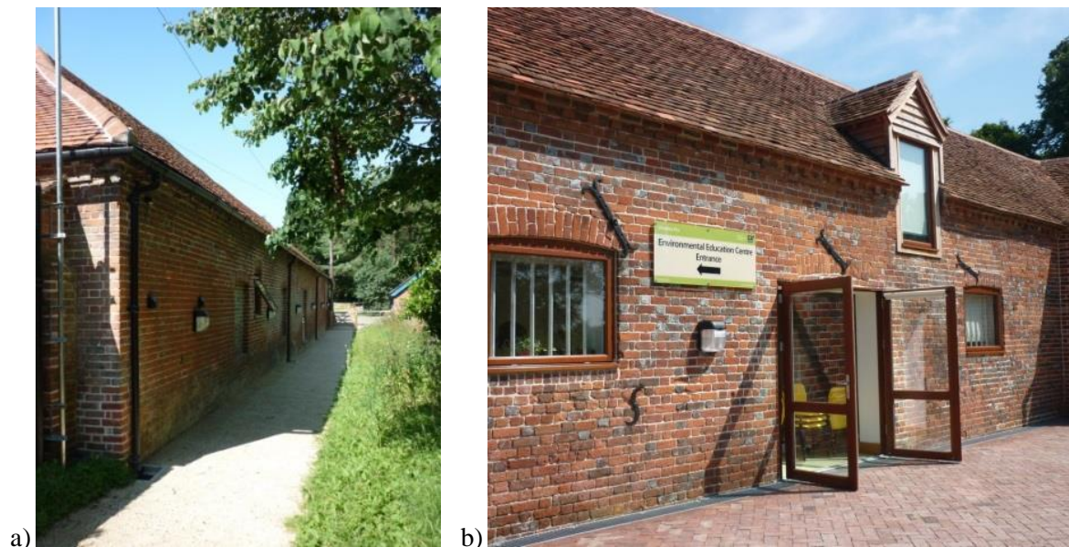
FIG 1. Building and external walls insulated a) north facing wall; b) south facing wall (access to teaching area)
