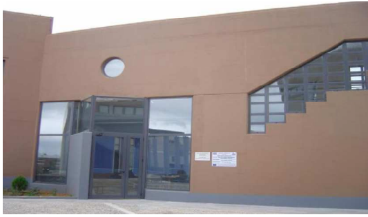
Figure 1. The Maintenance support building of the Technical University of Crete.
