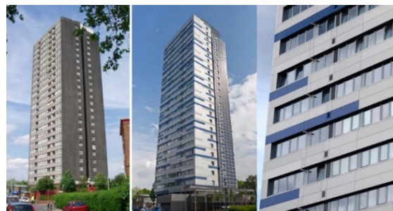
Figure 1 Ferrier Point, pre- and post-refurbishment
