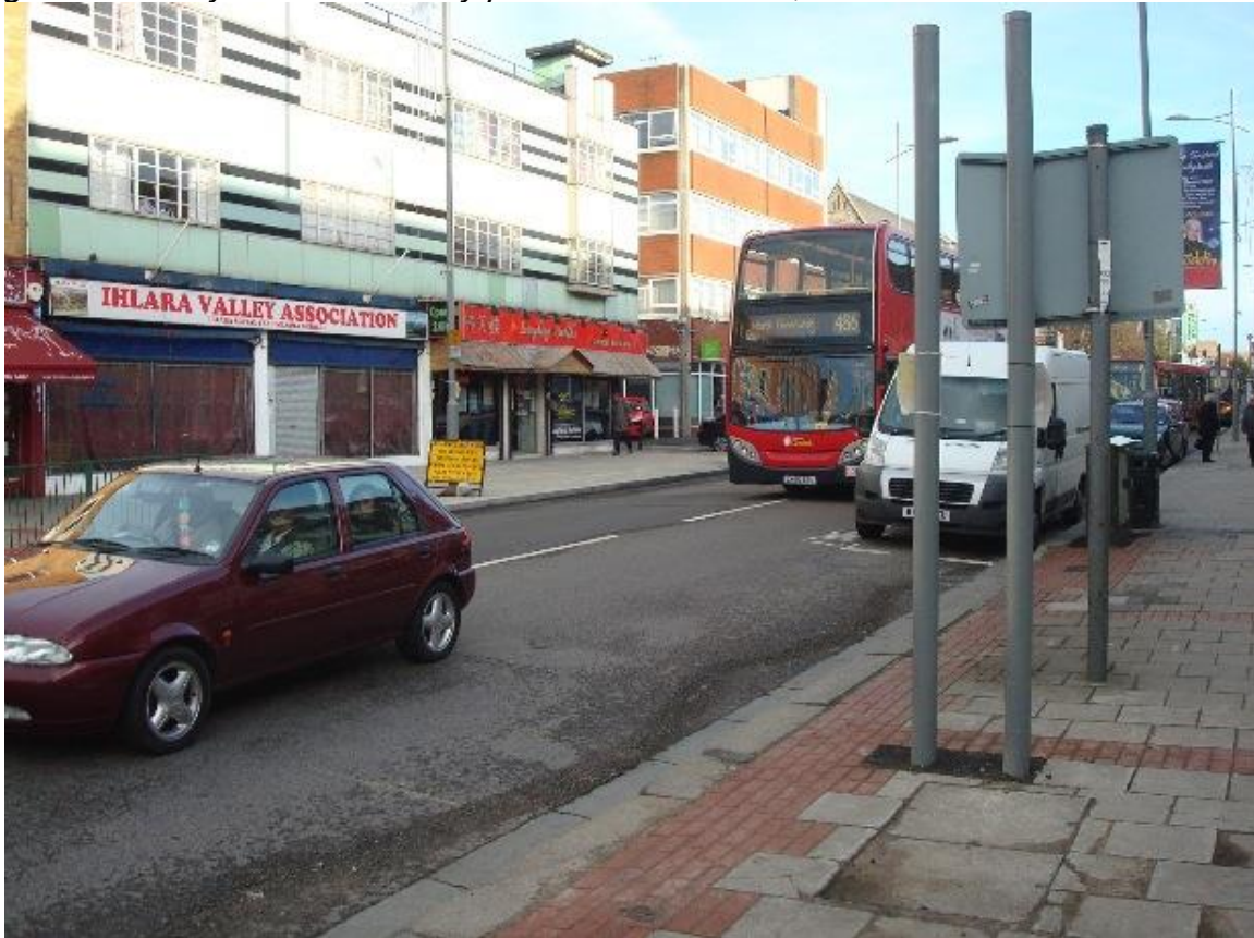
Figure 4: Bexleyheath Broadway prior to construction, November 2012
