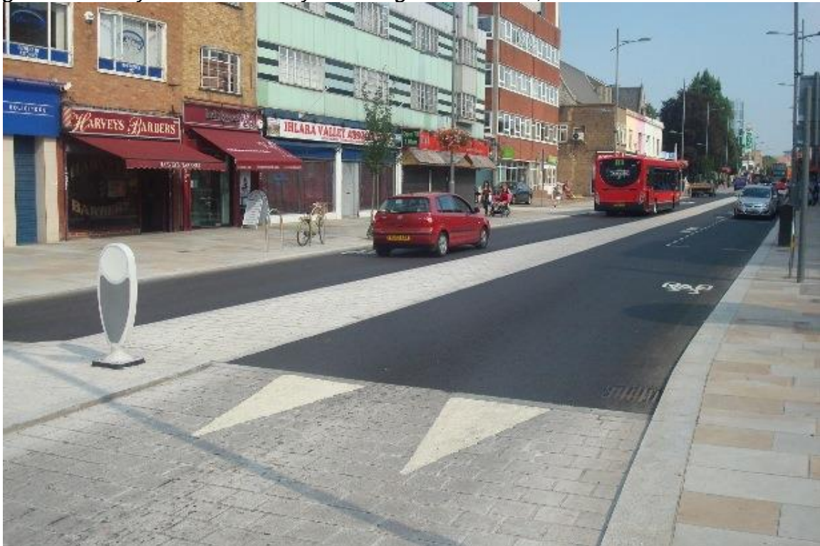
Figure 5: Bexleyheath Broadway following construction, June 2013
