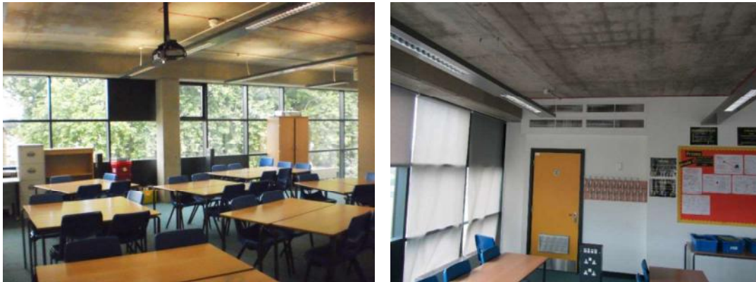
Figure 4.16. Internal view of a typical classroom with exposed ceiling and one operable window (left), the outlets for mechanical ventilation (right)
