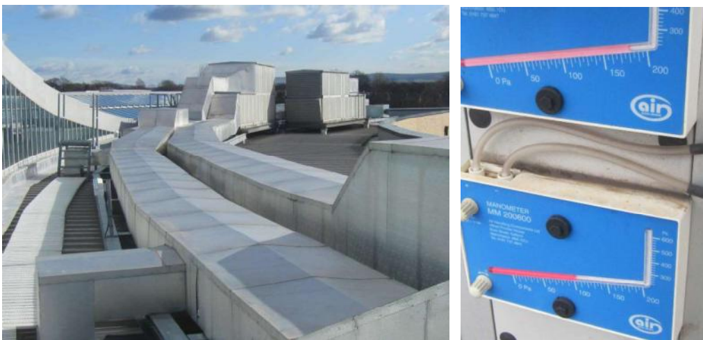
Figure 8.7. Mechanical ventilation system in Building A: sharp bends and high aspect ratios increase system pressure drop and specific fan power (left), system pressure drop will even further increase if air filters pass their recommended final pressure drop.
