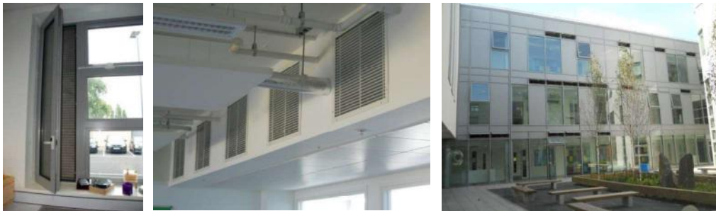
Figure 4.12. Cross ventilation strategy for Building D: operable windows (left), plenum air intake (middle), and motorised vents on the corridor side (right)
