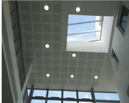
Figure 7.14. Thermal triggers for stack ventilation in the atrium space had not been programmed in Building D.
