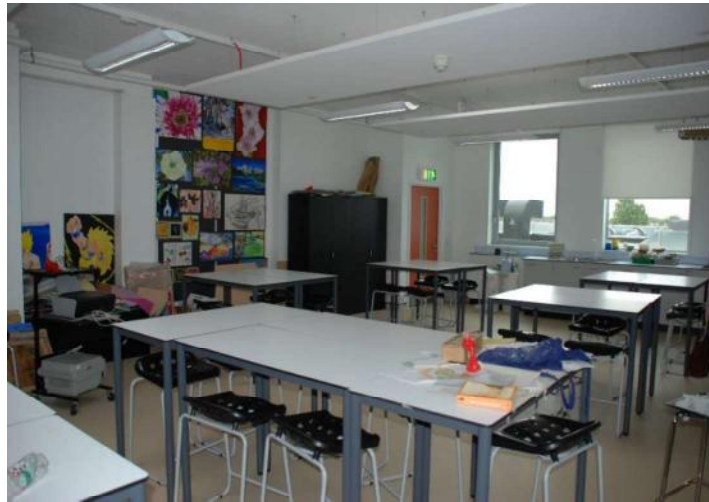
Figure 6.25. Acoustically absorbing material and suspended acoustic rafts are used to control reverberation in Building D
