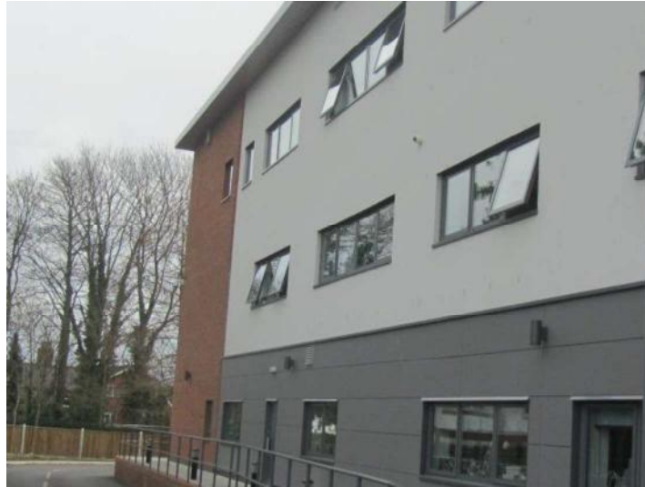
Figure 7.8. Top-hung windows in Building B: a number of windows were frequently open regardless of the mechanical ventilation strategy and external noise levels.
