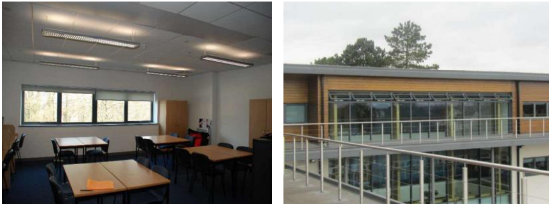
Figure 4.6. Internal view of a seminar room with ceiling mounted radiant panel (left), the motorised vents in the atrium are open to reduce CO 2 levels (right).
