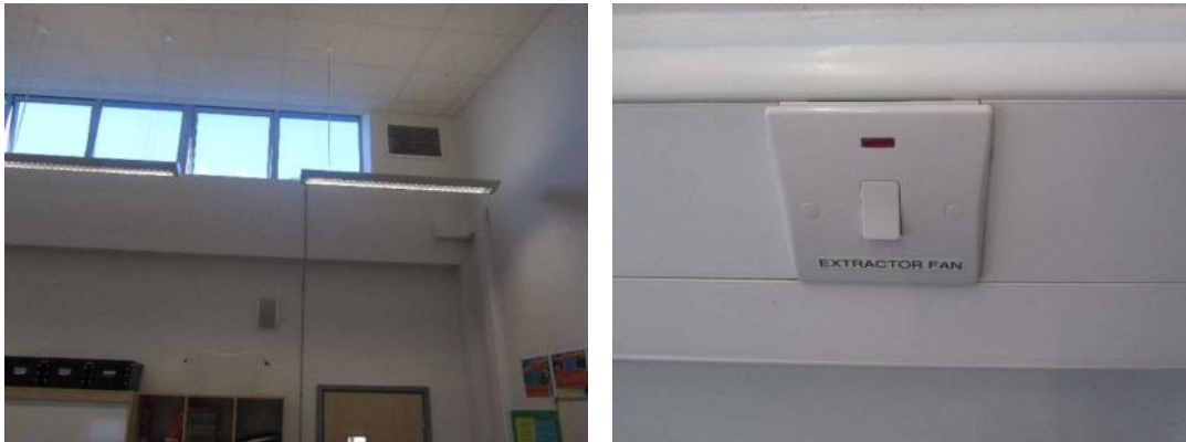
Figure 4.9. Ventilation strategy in Building C: manually operable clerestory windows and extract fans enable cross/stack ventilation in classrooms (left), extract fans are activated by a manual switch if teachers feel ventilation has to be improved (right).
