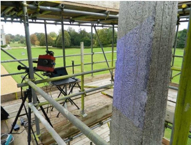
Figure 7: ATOS 3D scanner on the scaffolding platform.
