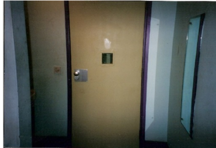
Figure 5: Watch panel on ward bedroom doors for indirect view of the bed through a mirror
