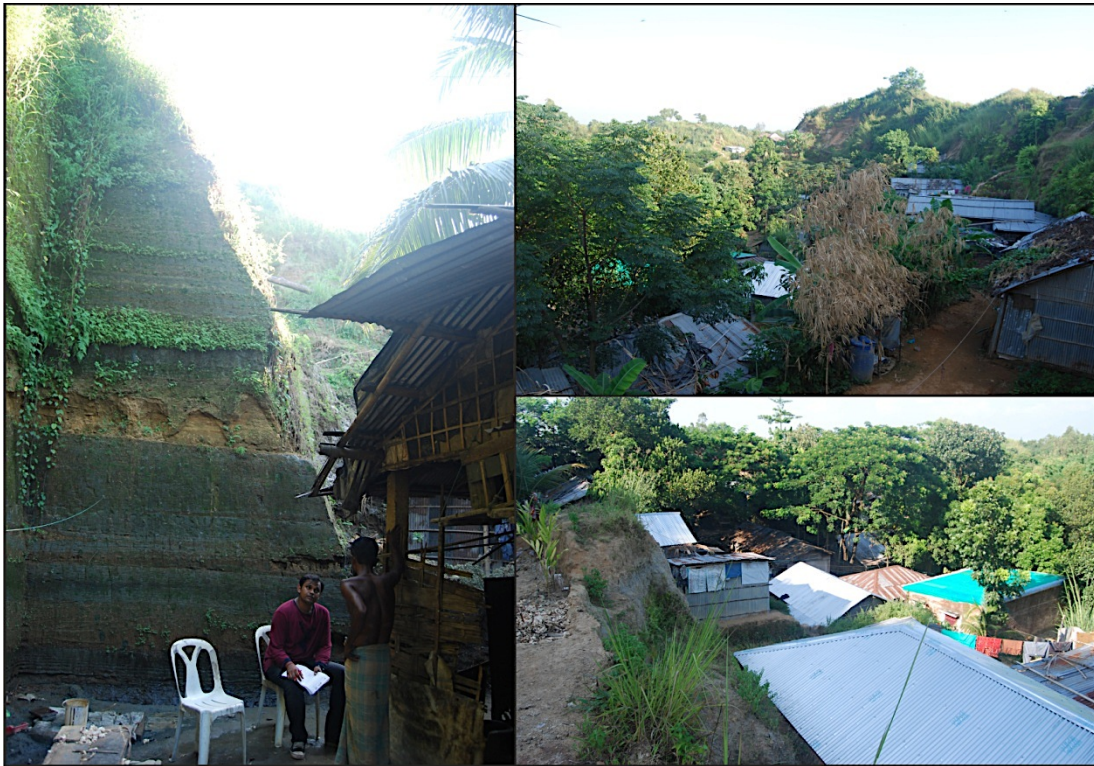
Figure 2. Photographs showing location of residential houses in dangerous hill slopes in Lighthouse Para, Cox's Bazar Municipality, Bangladesh. Source: Bayes Ahmed, 2014.
