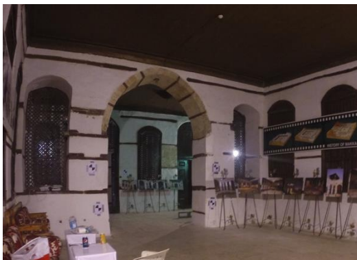
Figure C , Arch in the ground level.
