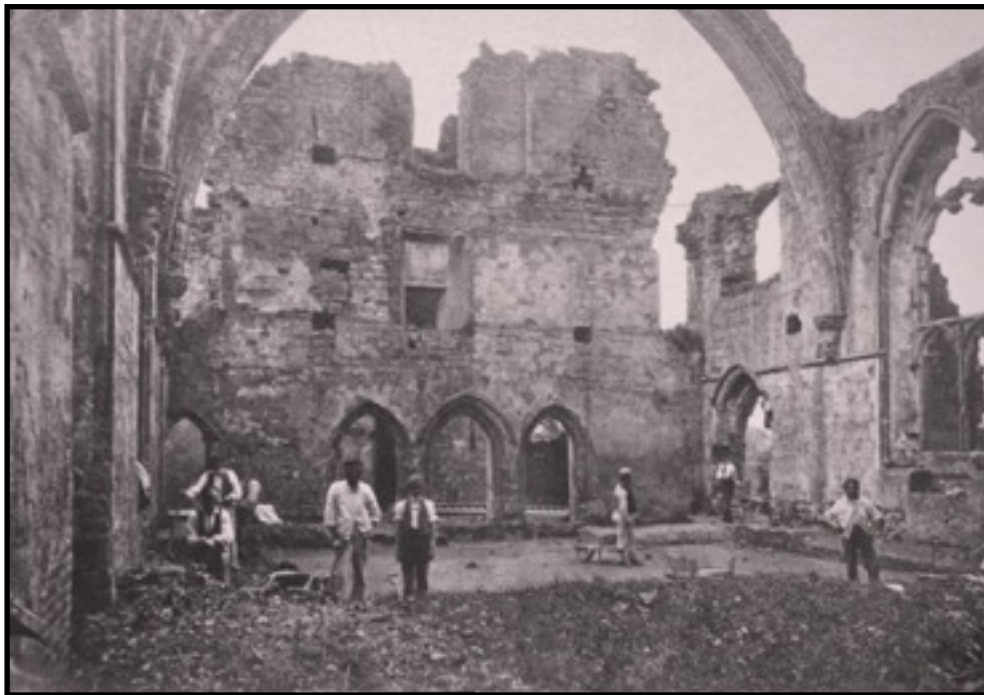
Figure 2 Builders at the site of the Old Palace, Mayfield c1864. Source: Archives of the Society of the Holy Child Jesus
