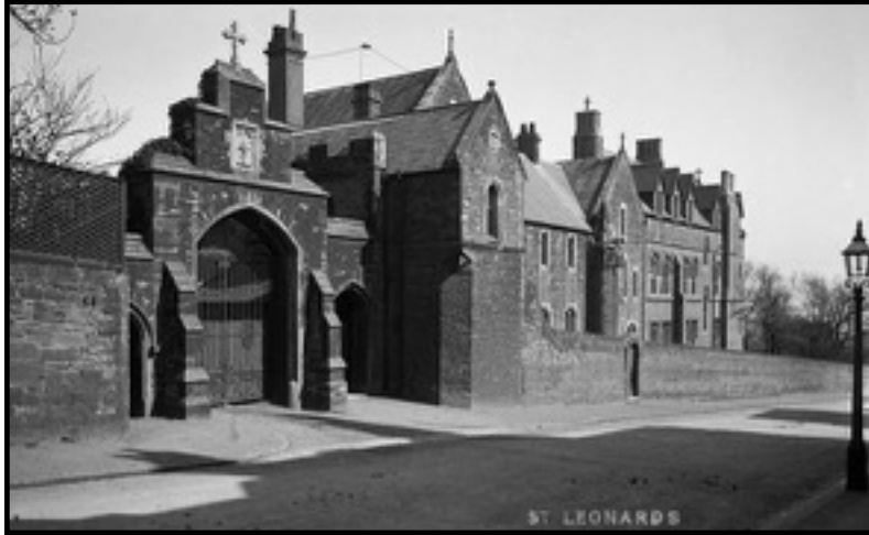
Figure 3.11 . Fig 3.13 Additions to St Leonards's convent by William Wardell, 1848 - 9. Source: East Sussex County Council
