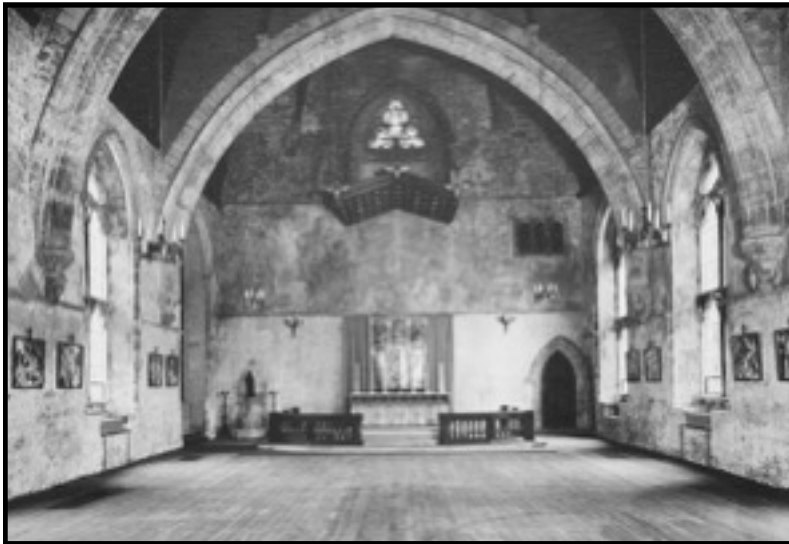
Figure 3.12. Interior of Mayfield chapel following restoration by Aelred Bartlett in 1951. Source: SHCJ Archive
