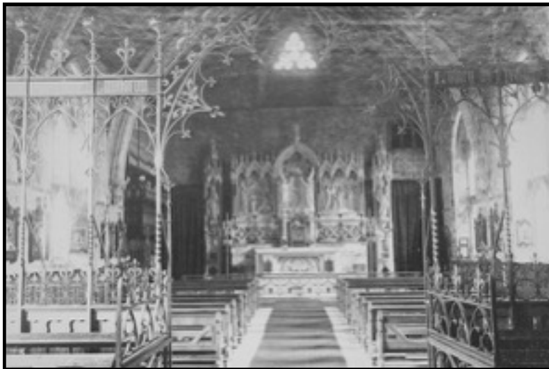
Figure 2.9 Chapel with addition of rood screen, reredos and rails by P. P. Pugin, 1881. Source: SHCJ Archives
