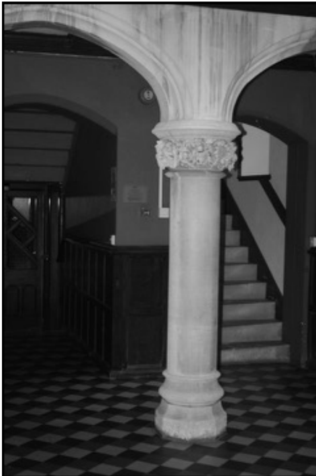
Figure 2.7 New staircase and interior by Goldie, 1873. Source: author
