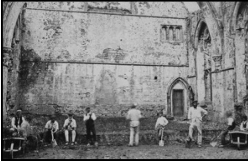
Figure 2.5. Workmen during the restoration of the former bishop's palace, c.1864. Source: SHCJ Archives
