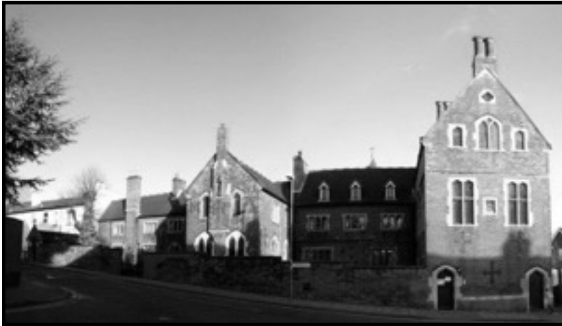
Figure 3.4 St Mary's Convent, Handsworth, 1840. Source: English Heritage
