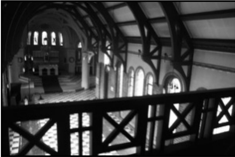
Figure 4.9. View of the interior of the Church of the Sacred Heart from the first floor nun's infirmary. Source: author
