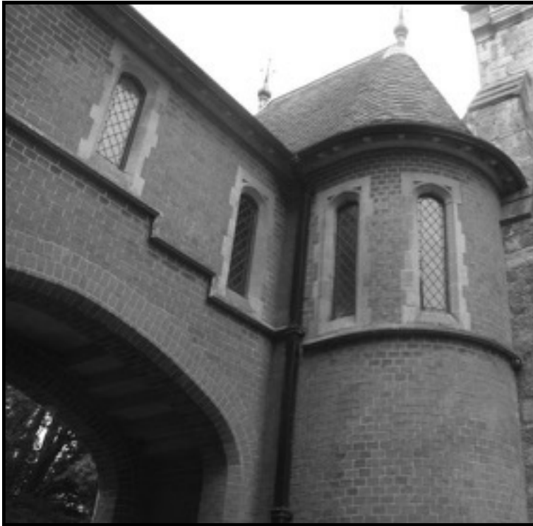
Figure 2.10 Gatehouse at Mayfield by P. P. Pugin, 1896. Source: author
