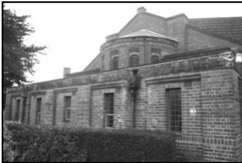
Figure 4.6. Church of the Sacred Heart Waterlooville, W. C. Mangan, 1923. Source: author
