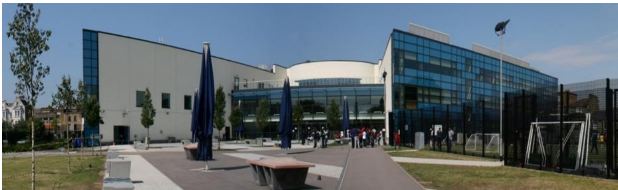
FIGURE 4. External view of Building B, south orientation
