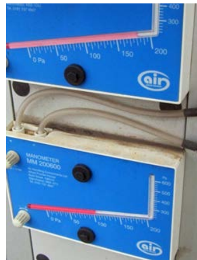
Figure 8: Building B ductwork installation with high aspect ratio and sharp bends (left). Dirty air filters further reduce the efficiency of the ventilation system (respective pressure drops shown in right).
