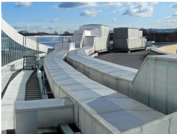
Figure 8: Building B ductwork installation with high aspect ratio and sharp bends (left). Dirty air filters further reduce the efficiency of the ventilation system (respective pressure drops shown in right).
