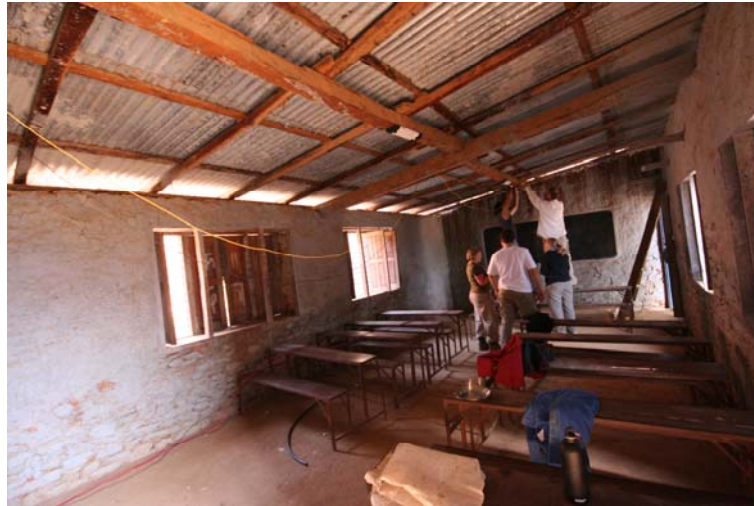
Fig. 9: UNSW team wiring up lights in one of the classrooms.
