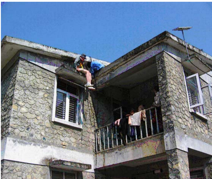
Fig. 1: Wiring being run from the PV panels on the roof of the health post Sankhe, Feb. 2004. The small panel visible in the upper right of the picture is used to supply power to the caretaker's home (not shown).
