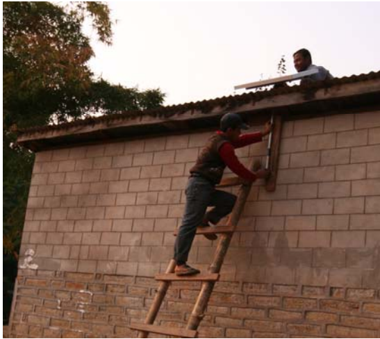
Fig. 11: Installation of one of the pole mounted PV panels.
