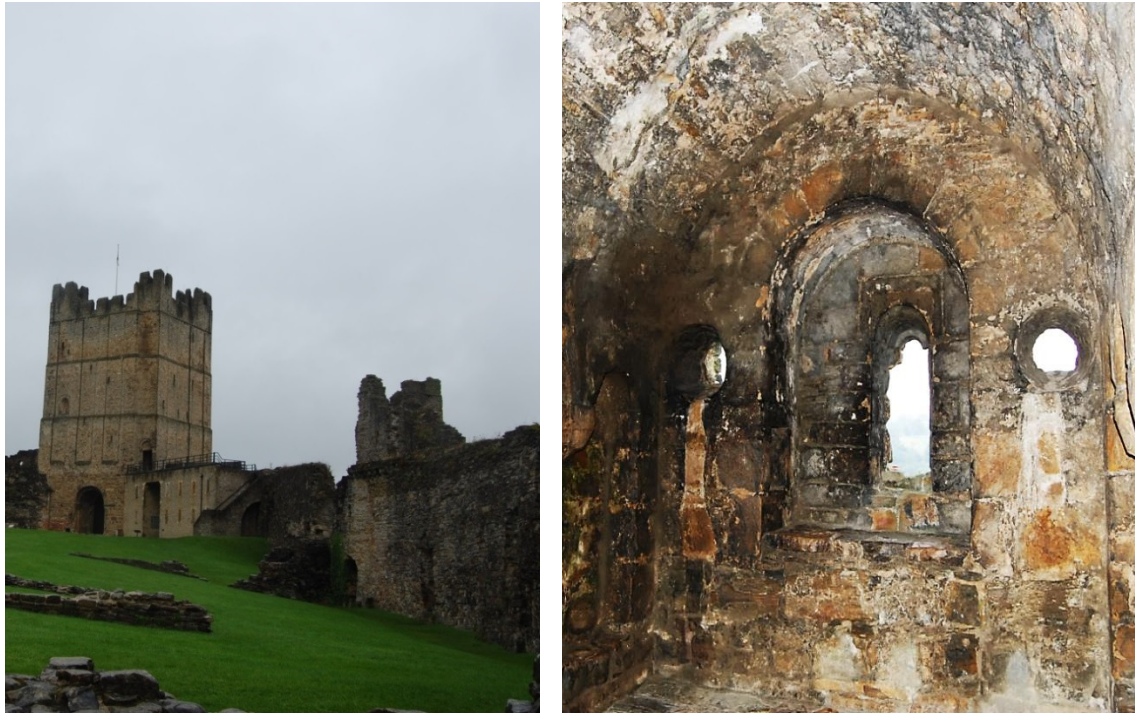
Figure 8.8. The Keep and Robin Hood Tower (left) and inside Robin Hood Tower, St. Nicholas's Chapel (right), Richmond Castle
