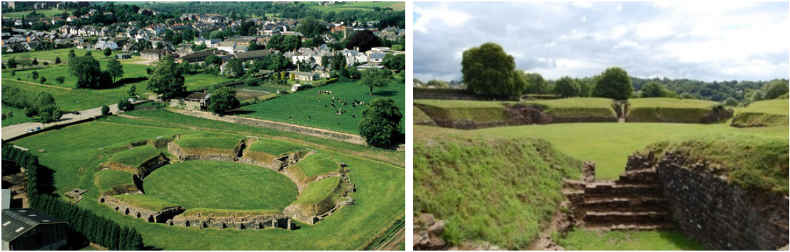
Figure 4.4. Aerial view of the amphitheatre, left (Cadw), and the amphitheatre from the ground, right
