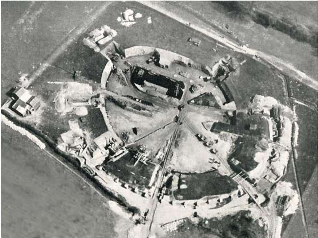
Figure 4.6. The excavation of the amphitheatre in the 1920s (Wheeler and Wheeler, 1928: Figure 2)
