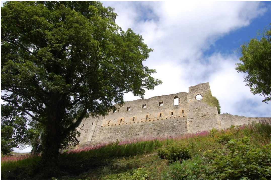
Figure 8.3. View of Richmond Castle from beside the River Swale
