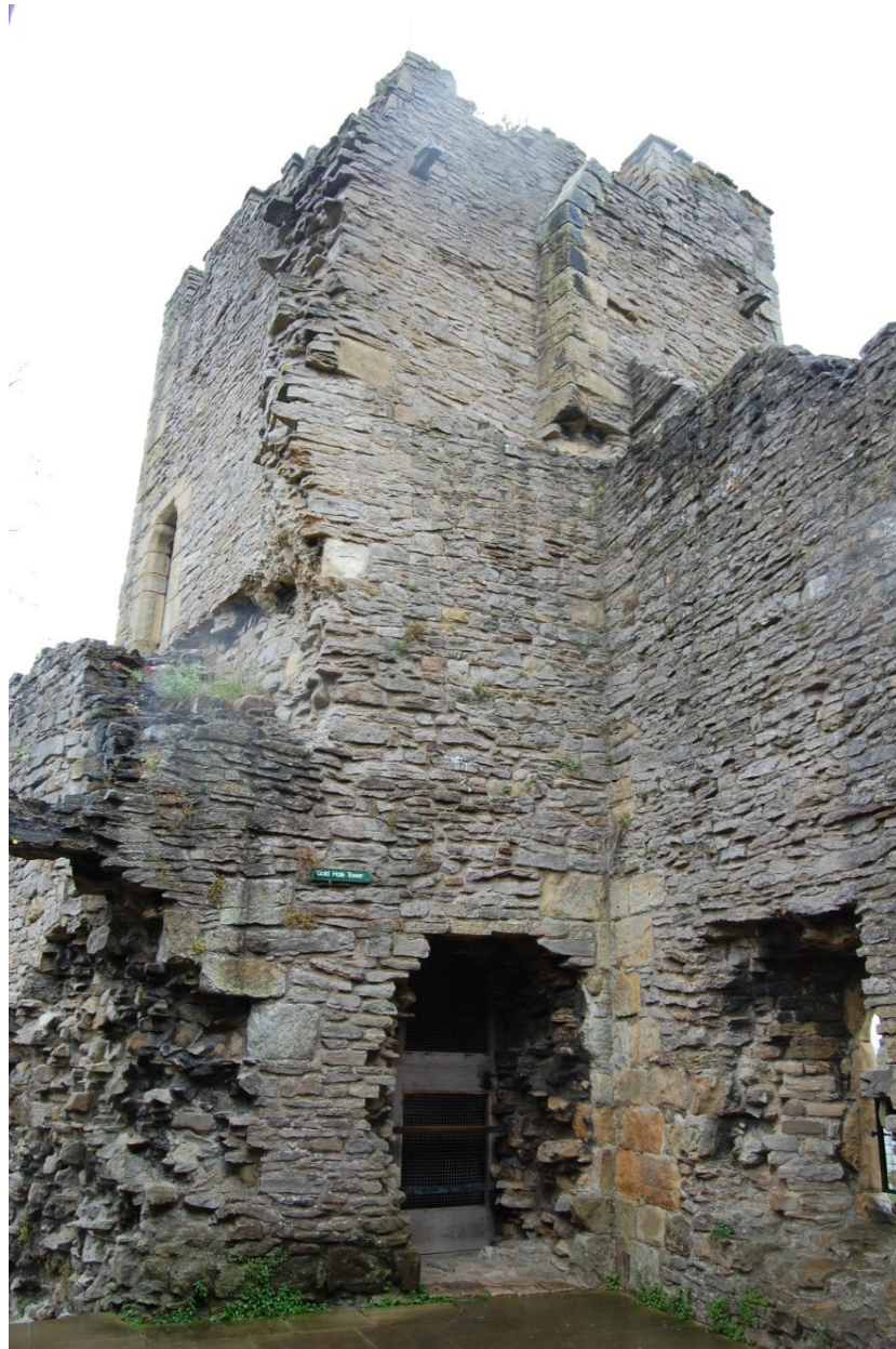
Figure 8.9. Gold Hole Tower, Richmond Castle
