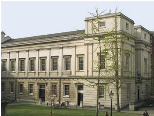
Figure 1 - Chadwick Building (North-East Façade)
