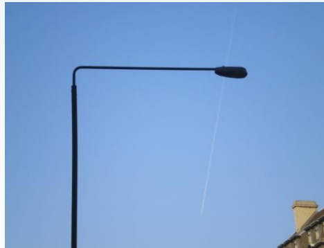
Street lighting – £1,600 each new or £450 for an upgrade
