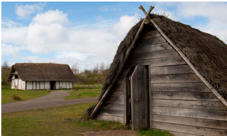
Figure 11 Reconstructed farm buildings at Bede's World Image © Bede's World.
