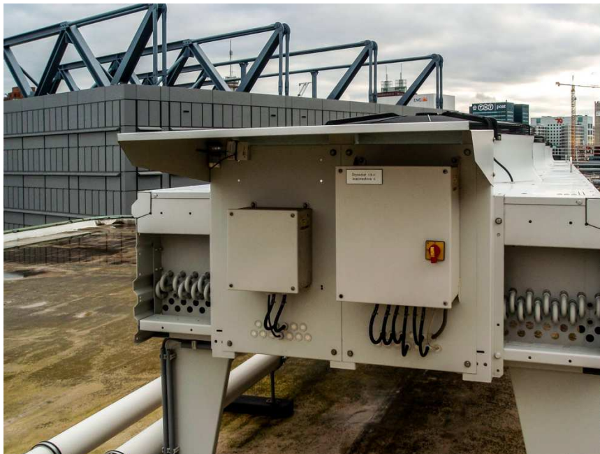
Figure 4.3: The roof terrace on the 9 th floor with air coolers.
