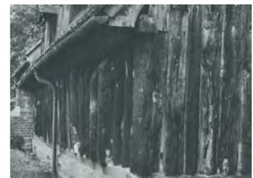
Figure 6: The short-baulk timbers of Greensted church built of oak and elm.
