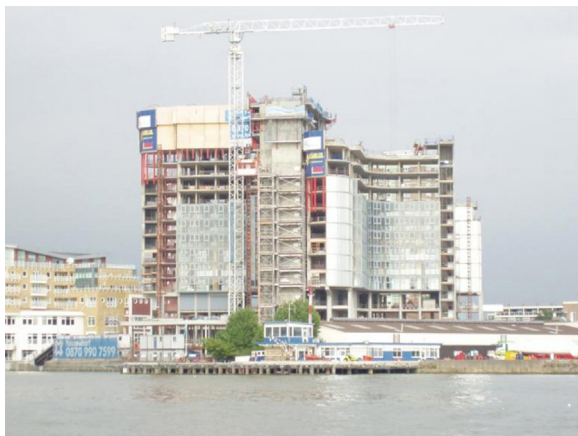
Picture 2. Falcon Wharf under construction. Source: Author.
