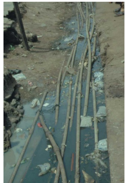
Figure 2. Open Sewer with Drinking Water Pipes Passing Through
