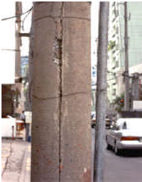
Figure 2.5: The corrosion of the steel reinforcement in this concrete power pole has cause it to split from end to end ( www.ingal.com.au/IGSM/06.htm )
