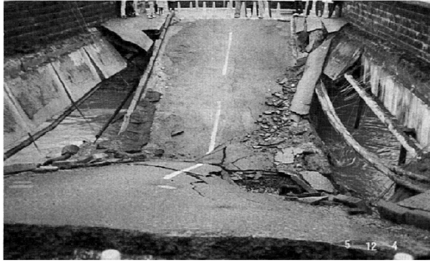
Figure 2.1: Collapsed Ynys-y-Gwas bridge [Woodward and Williams, 1988]
