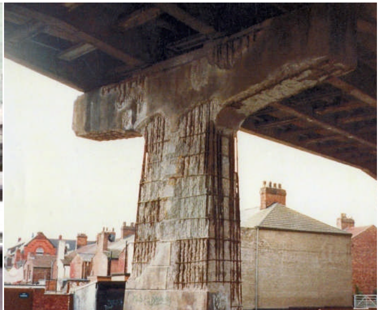
Figure 2.6: Severe spall and corrosion of the reinforcing steel on the retaining wall [P. Lambert & C. Atkins, 2007]
