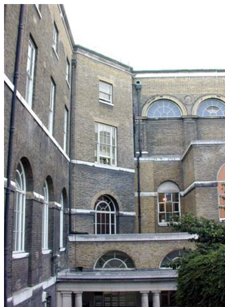
Fig. 20 - Richardson rebuilt the junction between the Wilkins building (right) and Donaldson's Library (left) and added the low level colonnade. Pale brickwork (top left) shows areas rebuilt after bomb damage
