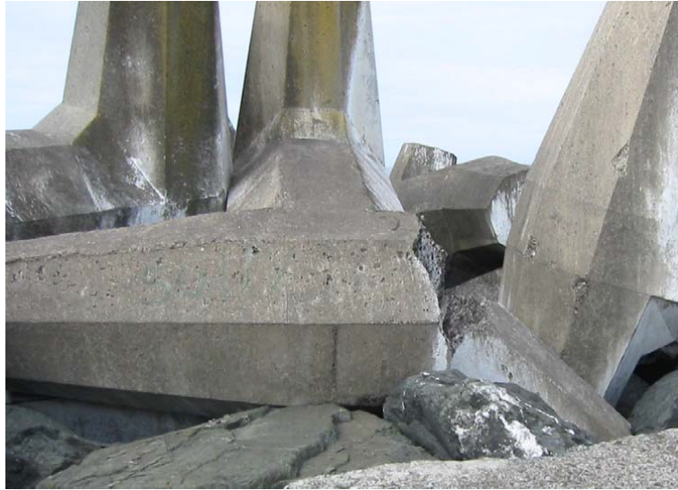
a. Example of fluke-stem fracture.
