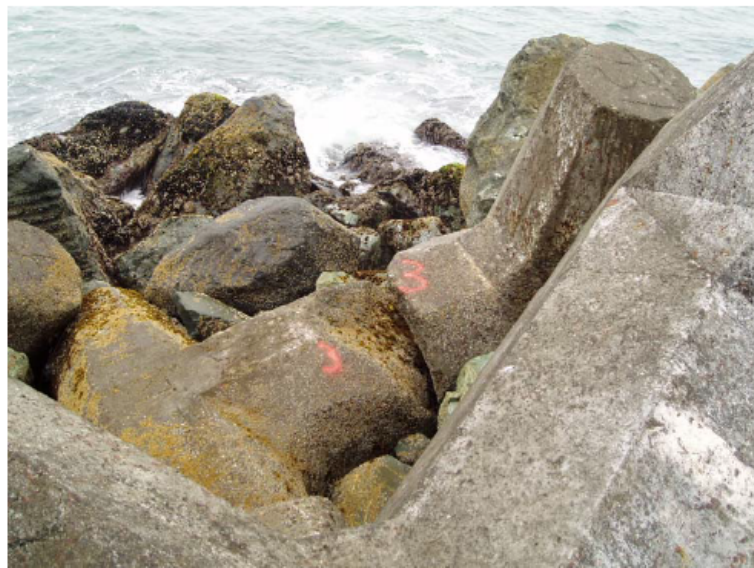
b. Example of middle-stem fracture.
