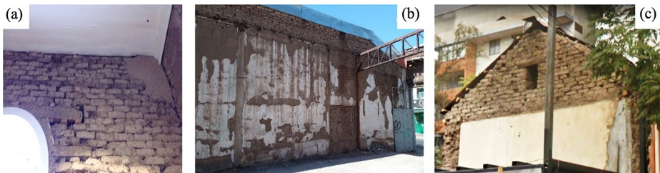
Fig. 6 Adobe masonry types in Barrio Yungay
