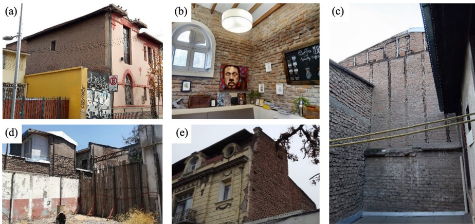
Fig. 5 Brick masonry types in Barrio Yungay
