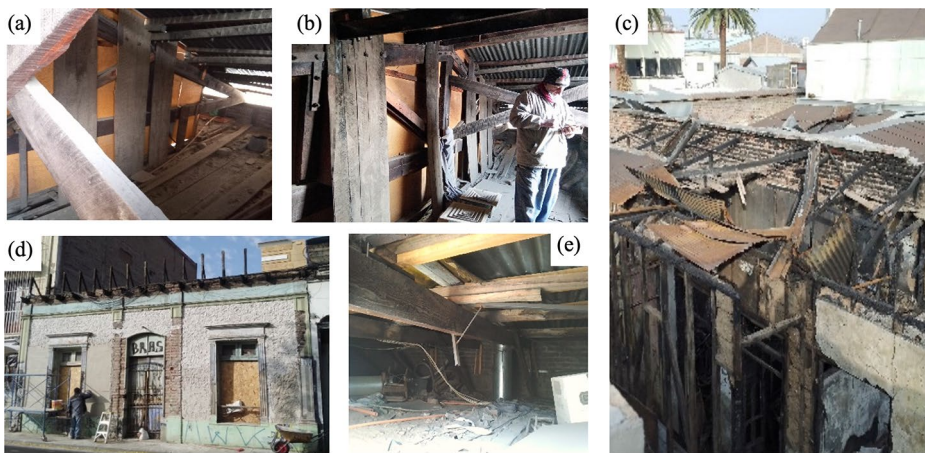
Fig. 7 Roof types: (a, b) timber trusses, (c, d, e) timber mono-pitch
