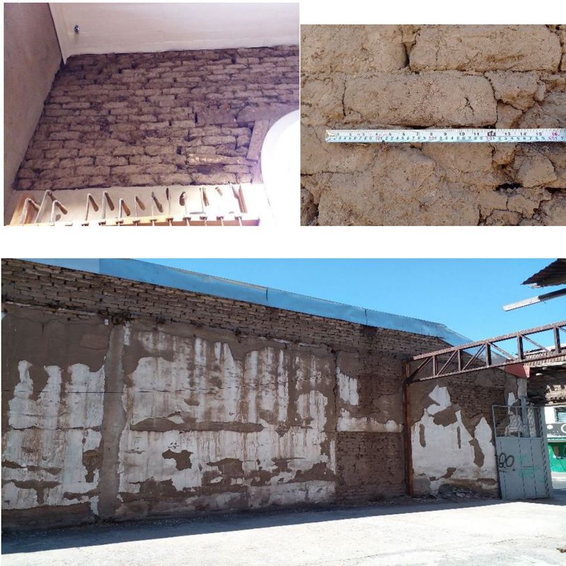
Fig. 22 Typical adobe masonry in the Yungay quarter
