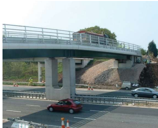
Figure 1: Mount Pleasant FRP-steel hybrid bridge during construction.
