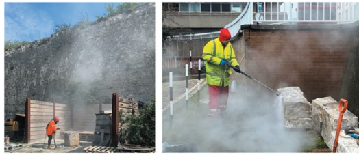
Figure 8. Left, sandblasting a stone to remove loose mortar. Right, jet washing a stone to clean it.
