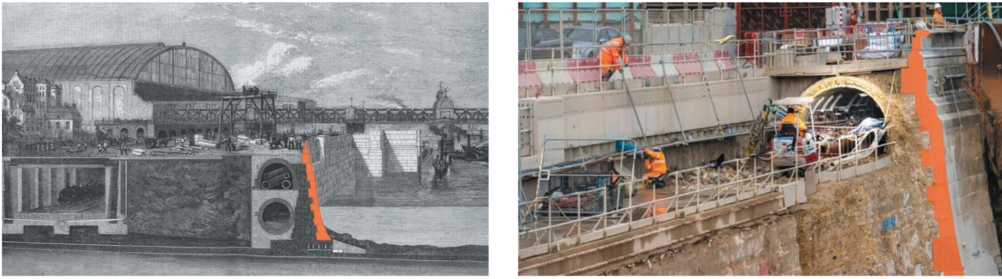
Figure 4. Left: Historic section through the newly constructed Victoria Embankment, June 1867, with the river wall highlighted in orange (Source: The Illustrated London News). Right: Image showing removal of a section of the river wall, highlighted in orange.
