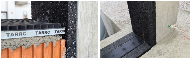
Fig. 3. Joints Type 1T and 1E (left) and Type 2 (right).
