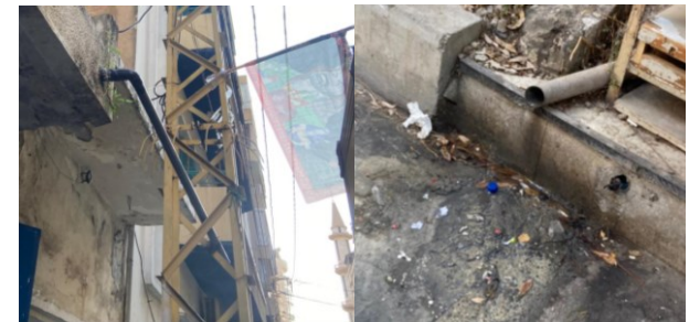
Image 14: Private drainage pipes spilling on sidewalk (Source: Basheer Itani)
