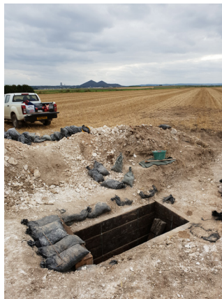
Figure 7.2 The original entrance to the tunnel complex known as ‘Mac’s Shaft’, re-engineered by the Durand Group. The famous ‘double crassier’ can be seen in the background. Source: author, Durand Group.
