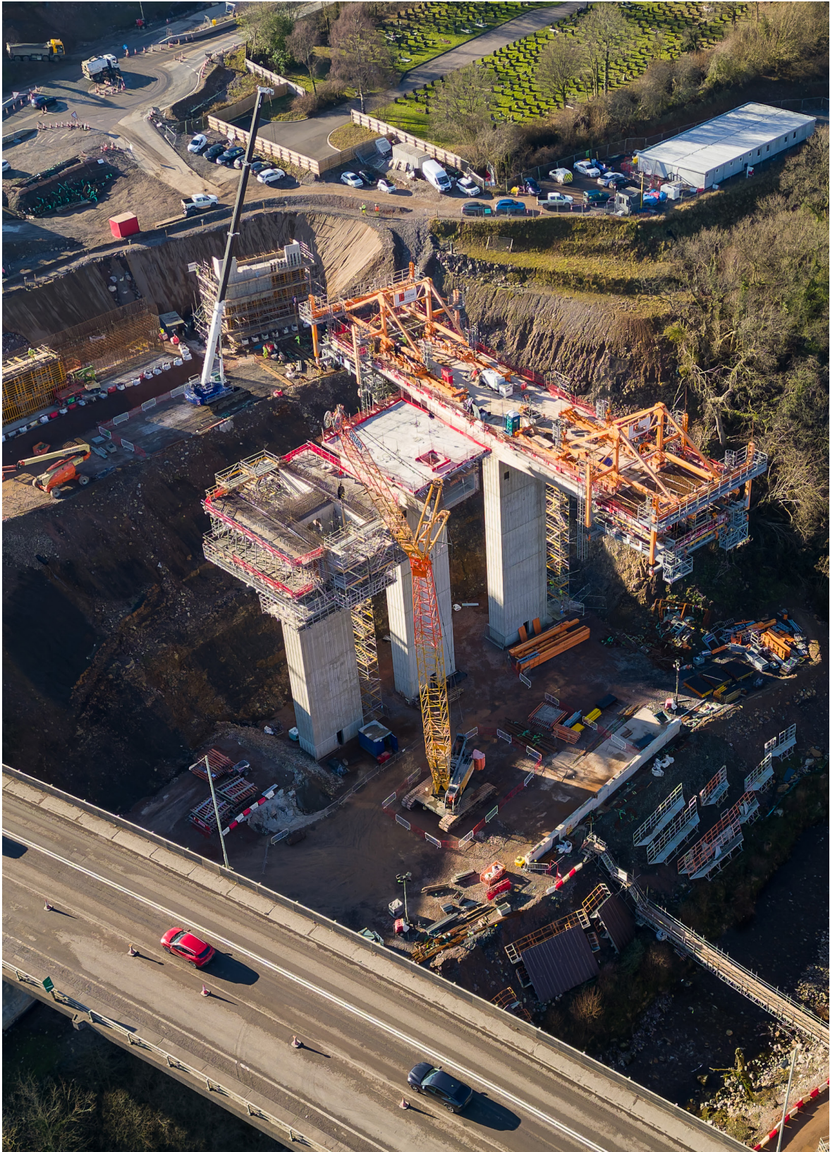
Image: Aerial view of bridge supports at a major road construction project in Wales (Heads of the Valley, Merthyr) ©WhitcombeRD / iStockphoto.com
