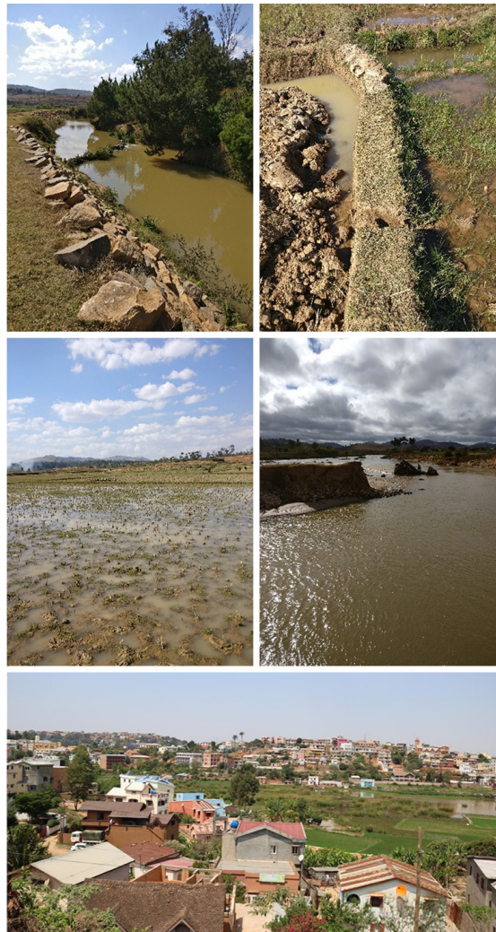
Figure 4 Top left: simple, wooden structure barrage on the Mambakely River. Top right: small, temporary water outlet between fields at Amparafara. Middle left: vast rice fields that were just inundated with water released from canal, on low-lying plains near St Paul's Theological College at Ambatoharanana. Middle right: larger-sized barrage at Antaramanana, built of earth and wood, part of it already eroded. Lower: valley and hillslope cultivation and urbanisation, Antananarivo
