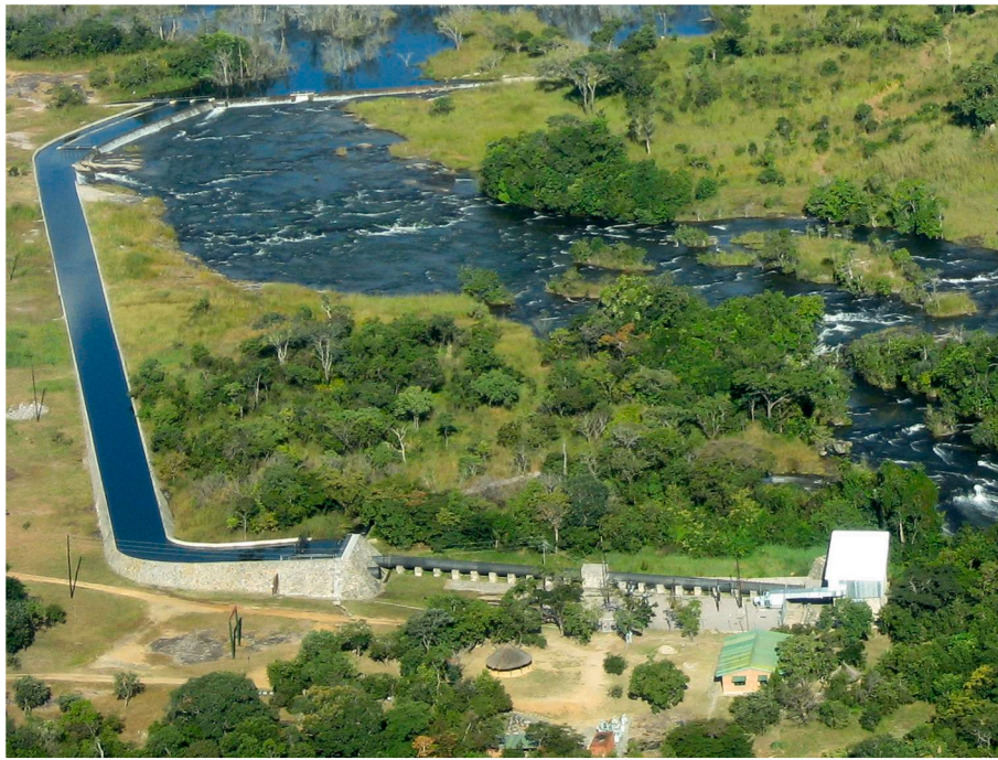
Fig. 6. Bird's eye view of the Zengamina hydropower scheme. Source: (North West Zambia Development Trust, 2013).
