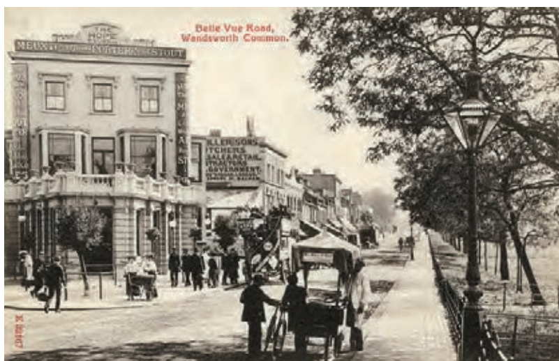
436. The Hope Tavern (of 1864–5, with later additions) and Bellevue Road in the early 1900s, looking south-west
