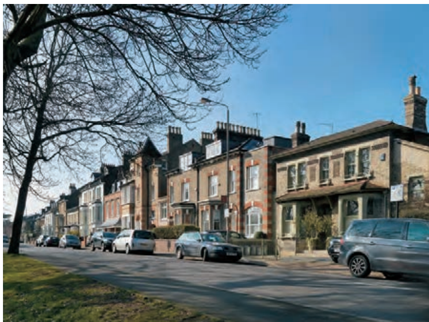
437. St James's Drive in 2013, looking south. In the foreground (right to left) No. 97, Nos 95 & 93, and No. 91 (with tower); Nos 75–89 beyond
