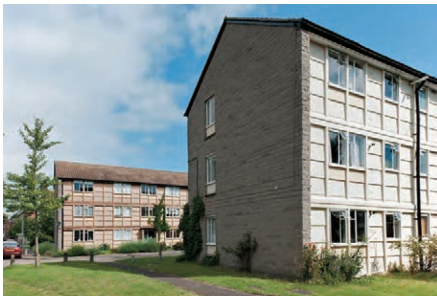
444. Post-war Cornish unit flats at 1–16 Mayford Close, looking north in 2012
