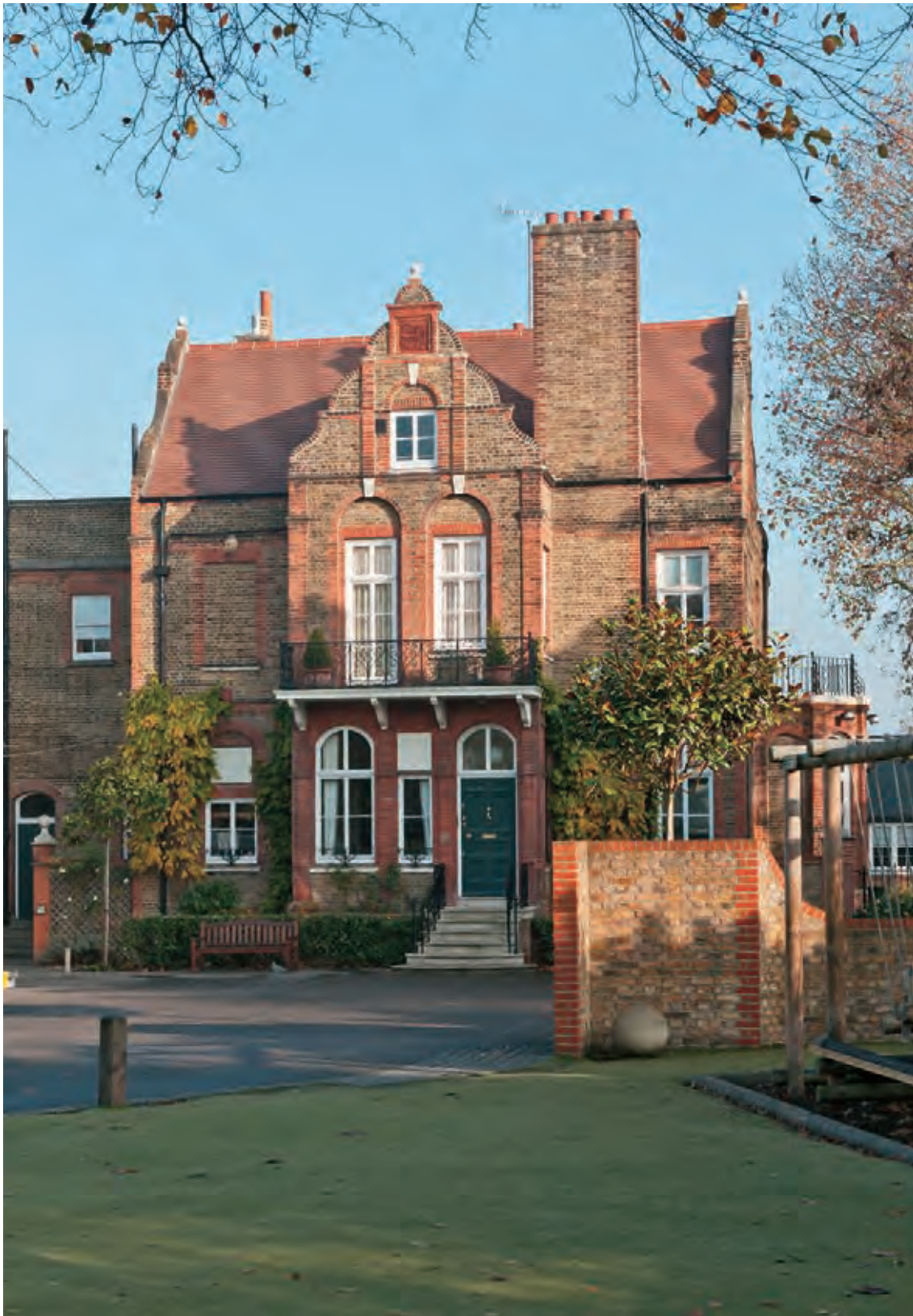
418. 26 Bolingbroke Grove (now Northcote Lodge Preparatory School for Boys) in 2011. E. R. Robson, architect, 1876
