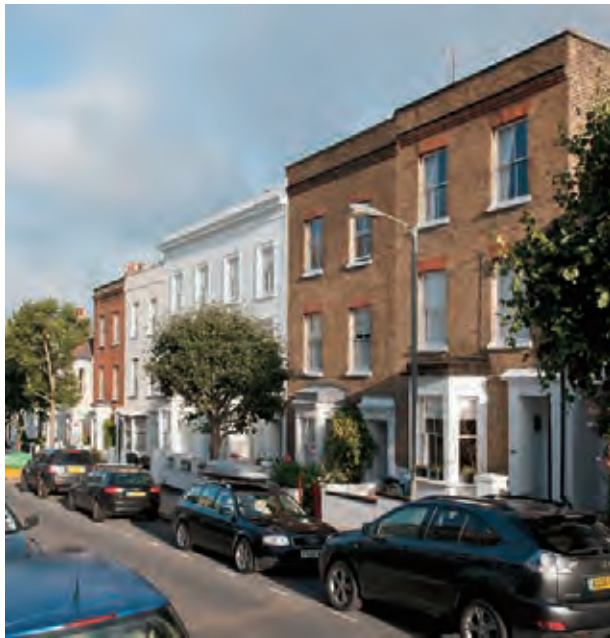
399. 99–109 Mallinson Road, 2012: typical early housing on the Conservative Land Society estate
