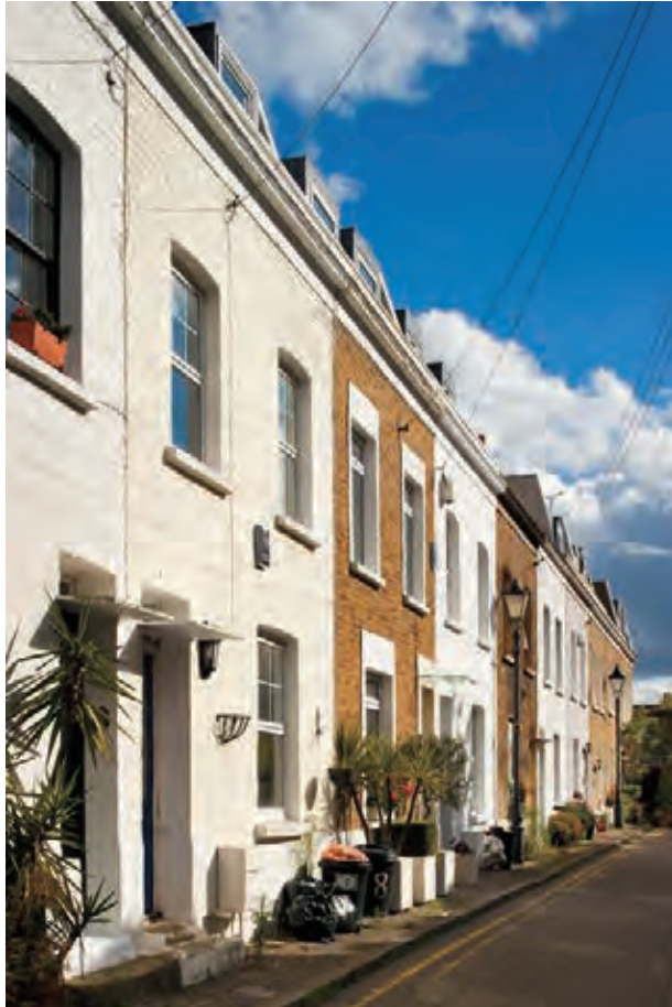
395. 6–15 Stonell's Road in 2012, looking south
