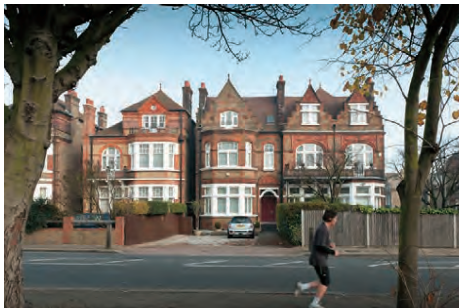
423. 14–16 Bolingbroke Grove, 2011. David Kettle, builder, 1883–7, possibly to designs by N. S. Joseph & Smithem, architects
