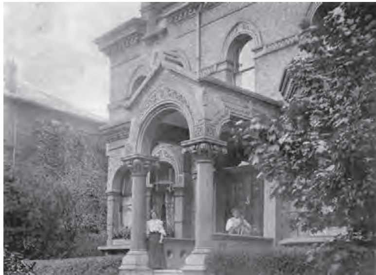
415, 416. Fairseat, 74 Nightingale Lane, elevation and floor plans. Rowland Plumbe, architect, J. J. Wilson, builder, c.1870–3 (opposite page), and entrance porch, 1902 (right)
