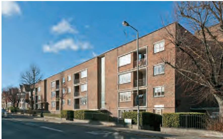
432. Abbott House, Nightingale Lane, in 2011. Battersea Borough Council, 1949–51
