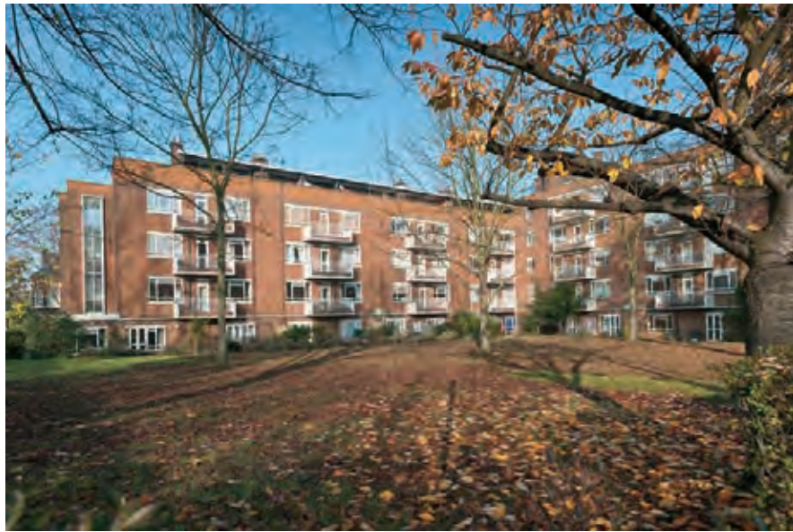
431. Stephen Sanders Court, Bolingbroke Grove, looking north in 2011. Battersea Borough Council, 1949–51
