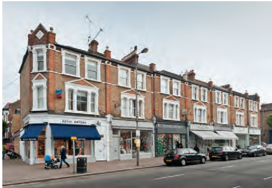
401. Shops at 133–145 Northcote Road in 2011
