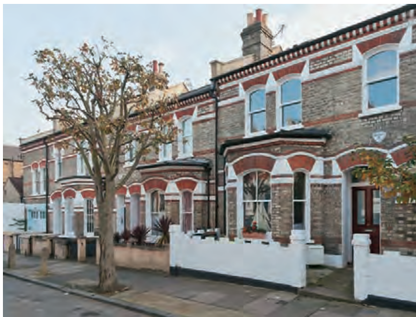
400. 68–72 Bennerley Road in 2011: characteristic Heaver houses, including his own and builder's yard at No. 72 (far left)
